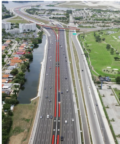
Modernization of 836 and XT lanes busway
