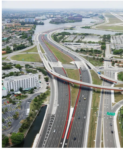
836 direct ramp to airport
